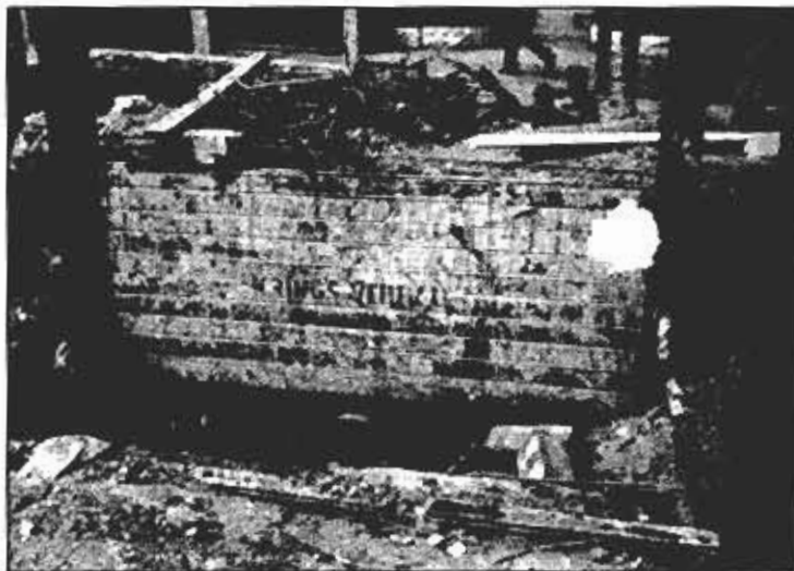
Shoring at the job site is typically vertical or horizontal heavy timber. Some contractors are using preformed metal panels, wales, braces, and shores. (Photos by author.)
