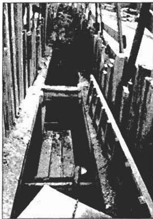
Shoring at the job site is typically vertical or horizontal heavy timber. Some contractors are using preformed metal panels, wales, braces, and shores. (Photos by author.)
