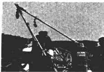
The specially designed Indian Wells Valley A-frame hauling system. Rescue personnel assemble the unit in about 15 minutes.
