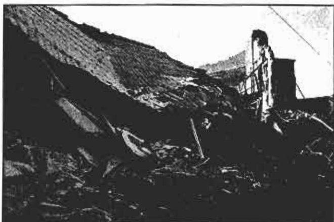
The snow load caused the collapse of each of these buildings. (Photos by John Norman.)
